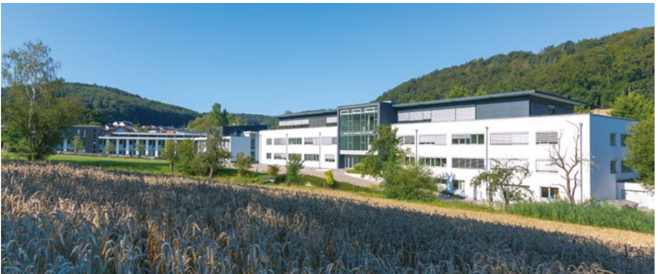
The company headquarters of REA Elektronik GmbH, 30 kilometers south of Frankfurt am Main, Germany
